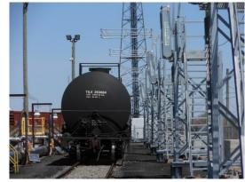
The solution had to be foundationless to avoid disturbing an existing stone wall. According to site personnel, the stone wall was well over 100 years old. Distributing the wall would have resulted in a lengthy and expensive permit process with no guarantee that they would be able to move forward. Benko Products custom designed a GREEN foundationless railcar platform as the solution. Benko mounted a common stationary platform to a skid with a concrete counterweight securing the station in place.
