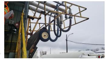
complicated to use. The truck station had three existing loading hoses on an existing platform. The client wanted a solution that would provide safe access and fall protection while allowing them to continue to use their current hoses.
